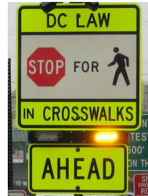
Rapid flashing beacon
