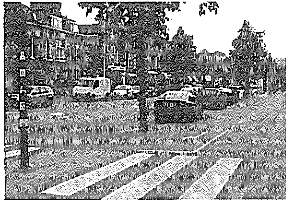
Figure 2 Example of Staging area for cycle track crossing
