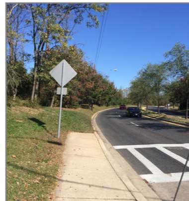
Disconnected/missing sidewalk between Edmonston Road and Breezewood Drive.
