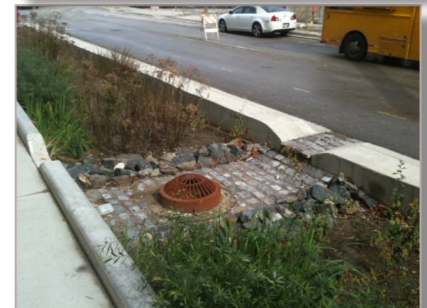
Top image: bioswale with a grassed strip along the edge. Bottom image: a narrower bioswale with inlets directing water from both the sidewalk (left side) and street (right side) into the treatment area.
