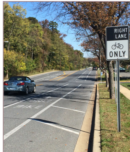
Bike lanes are present along both sides for the majority of the roadway. This report recommends adding bike lanes where they are not currently present and adding features that enhance bike safety.
