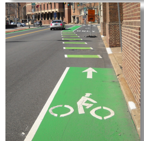
Examples of bike lanes striped (top) or covered (middle and bottom) with green retro-reflective thermoplastic to increase the safety of cyclists. Dashed areas indicate where vehicles may cross over.
