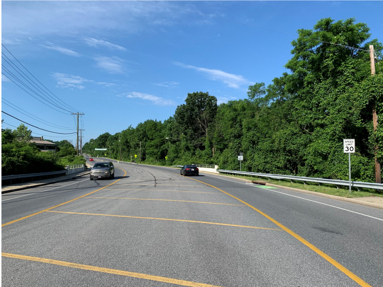
Looking towards Cherrywood Lane from roundabout at Cherrywood Ln and Greenbelt Metro Dr
