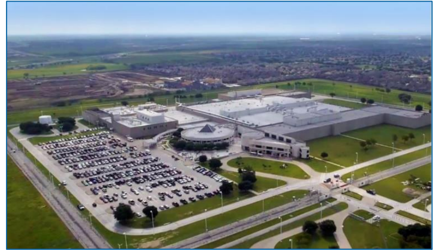
Texas Facility (constructed 1990)
