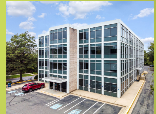
Nationwide Building Greenbelt Submarket 9111 Edmonston Rd Greenbelt, MD 20770 Property Manager Lincoln Property Company
