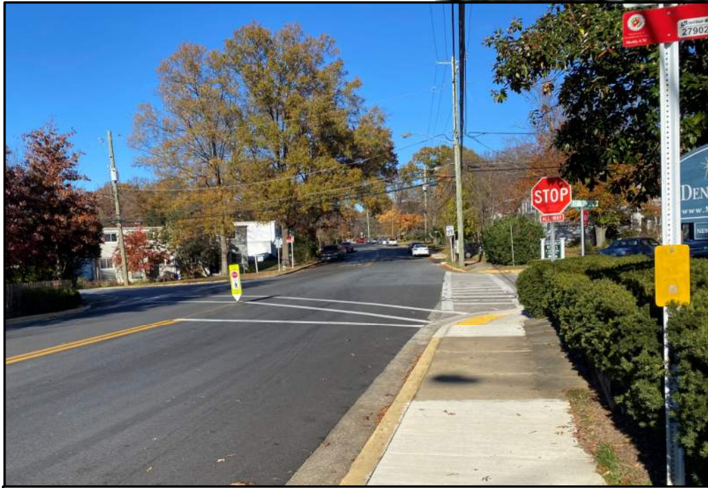
Existing crosswalk offers poor visibility and skewed alignment
