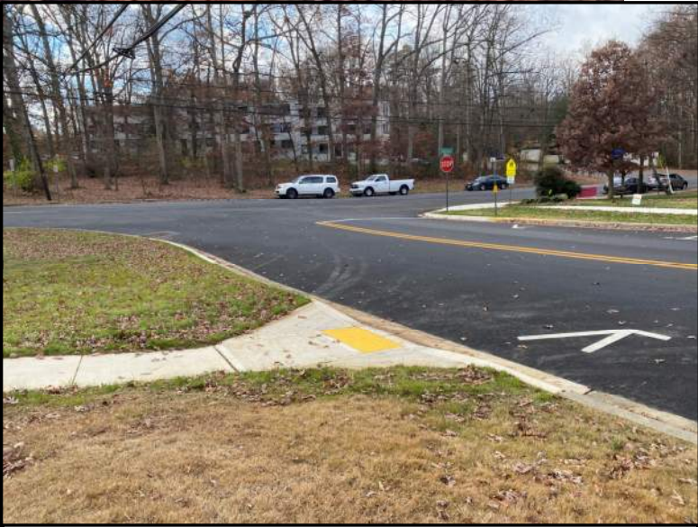
Existing ramp lacks connection to mid-block or intersection crossing
