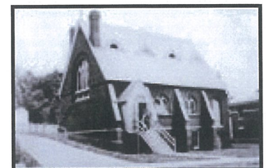
Pinckney Memorial Church. The remaining front wall will be part of the ATHA space.
