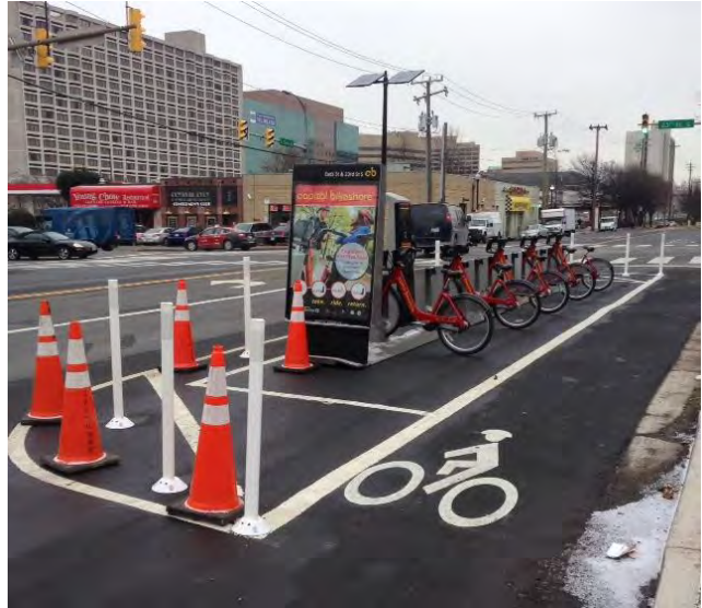
Figure 28: Protective buffer for Capital Bikeshare station in Arlington County, VA (Photo Credit: Euan Fisk Flickr)
